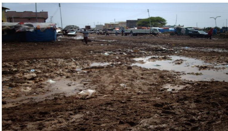
Figure 6: State of the Togwajale-Berbera road during wet season
